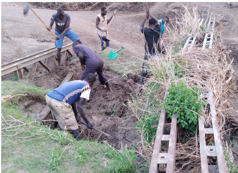
Digging out grates from old, buried bridge
