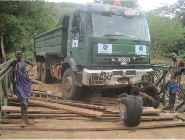
Large Lorry Stuck on bridge where grates are missing.
