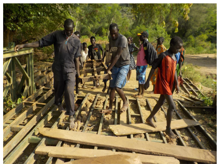
Replacing metal grates on damaged Kuron River Bridge
